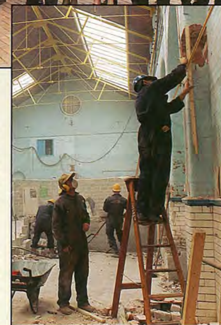
Refurbishment is underway at the Hoylake training centre in preparation for the new Powerlearning facility.
