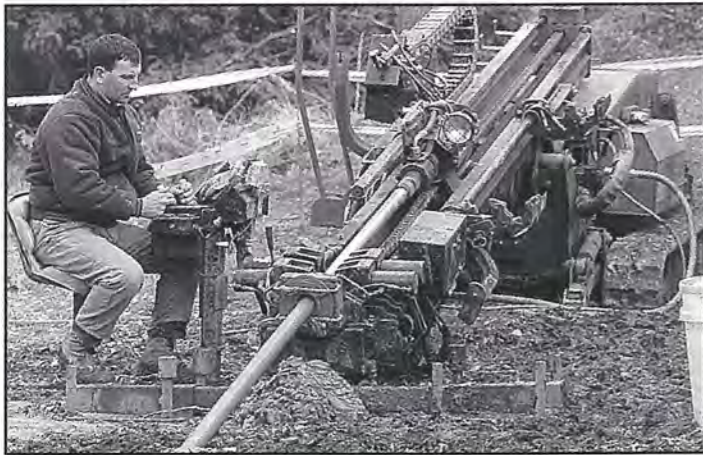
The special boring rig in action drilling steel rods under the River Dee to create a five inch bore hole.
