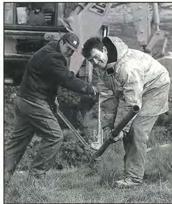
Members of the cable installation team pull rods back during the pre-reaming.
